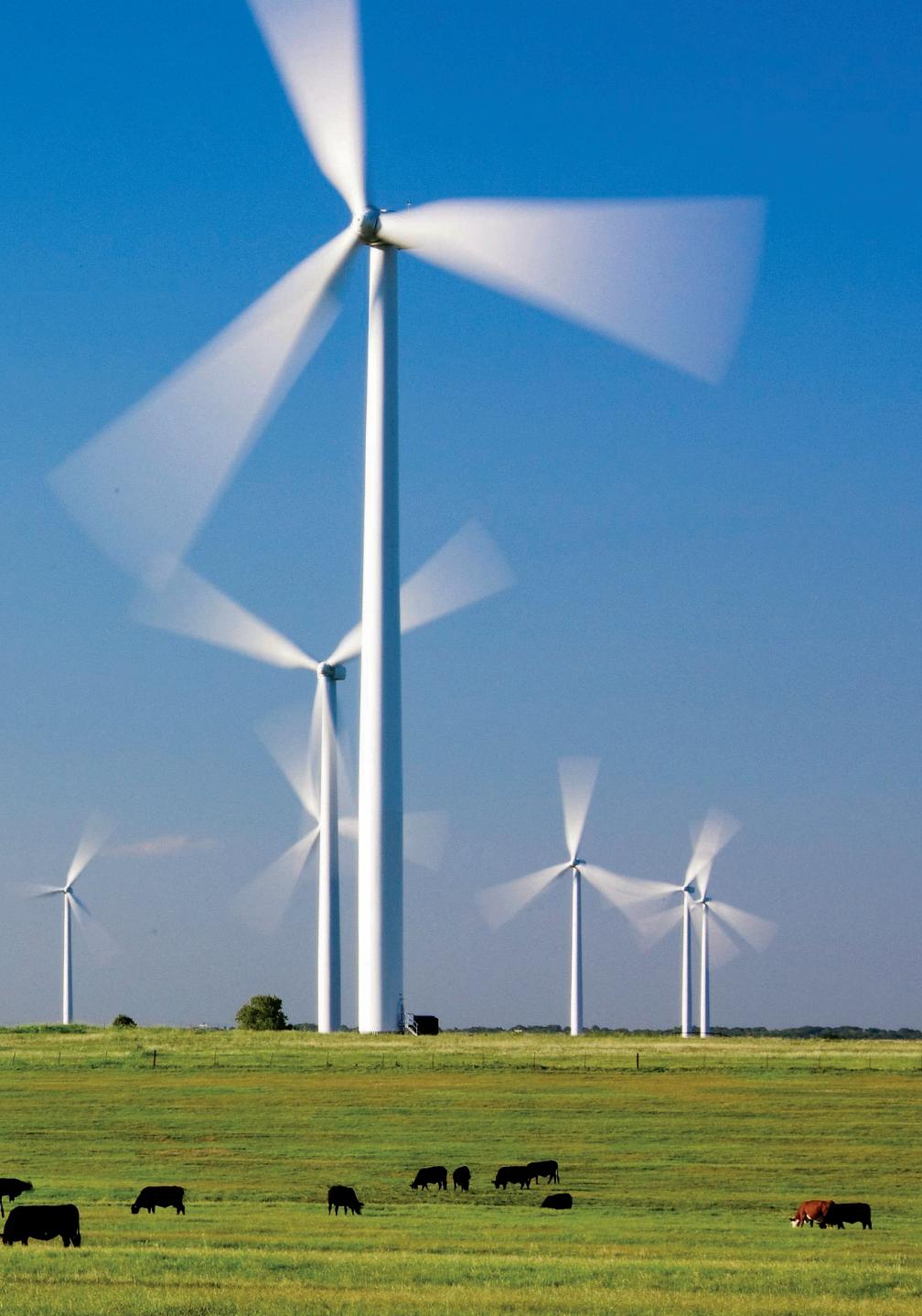
Wind turbines near Muenster, Texas. In 2015, wind power made up 12% of electricity production in Texas.
